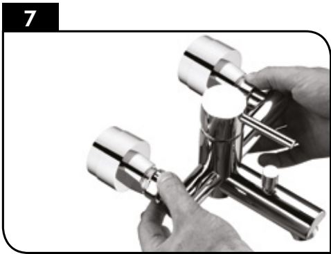
7 Approach the tap to installation and directing the eccentrics couplings in line with the nuts of the tap. Screw nuts with hands on eccentrics couplings.
